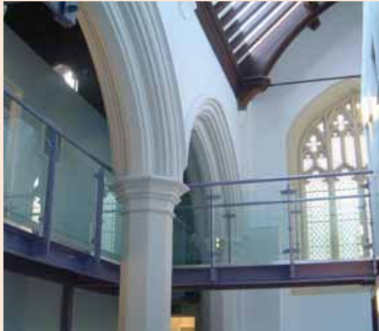
St John's Church, Hafod, Swansea
